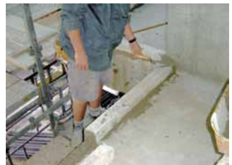
Ultralintel being bonded to create the hob.
