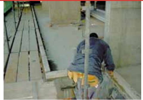
Hob being bonded to slab edge.
