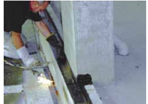
Waterproofing membrane being formed.
